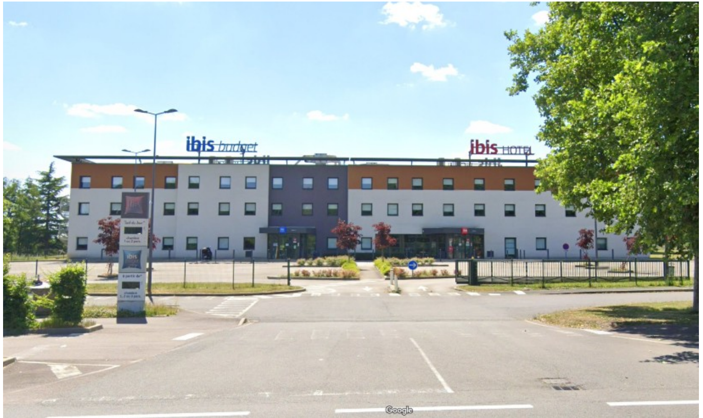
Das Hotel Ibis in Montceau-les-Mines
